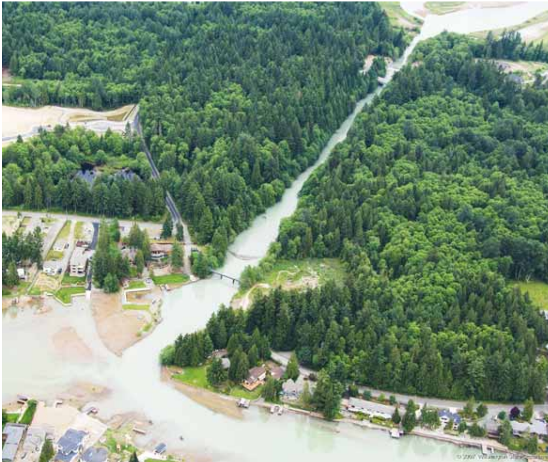
Exhibit 9. View of the Printz Basin Flume looking east. Printz Basin is visible in the distance.
