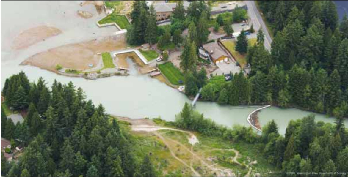
Exhibit 10. View of the Printz Basin Flume as it flows into Lake Tapps.
